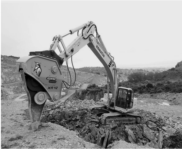
Fig. 1. XR 42 vibration ripper from Xcentric Ripper in an open-pit mine [L. 2]
